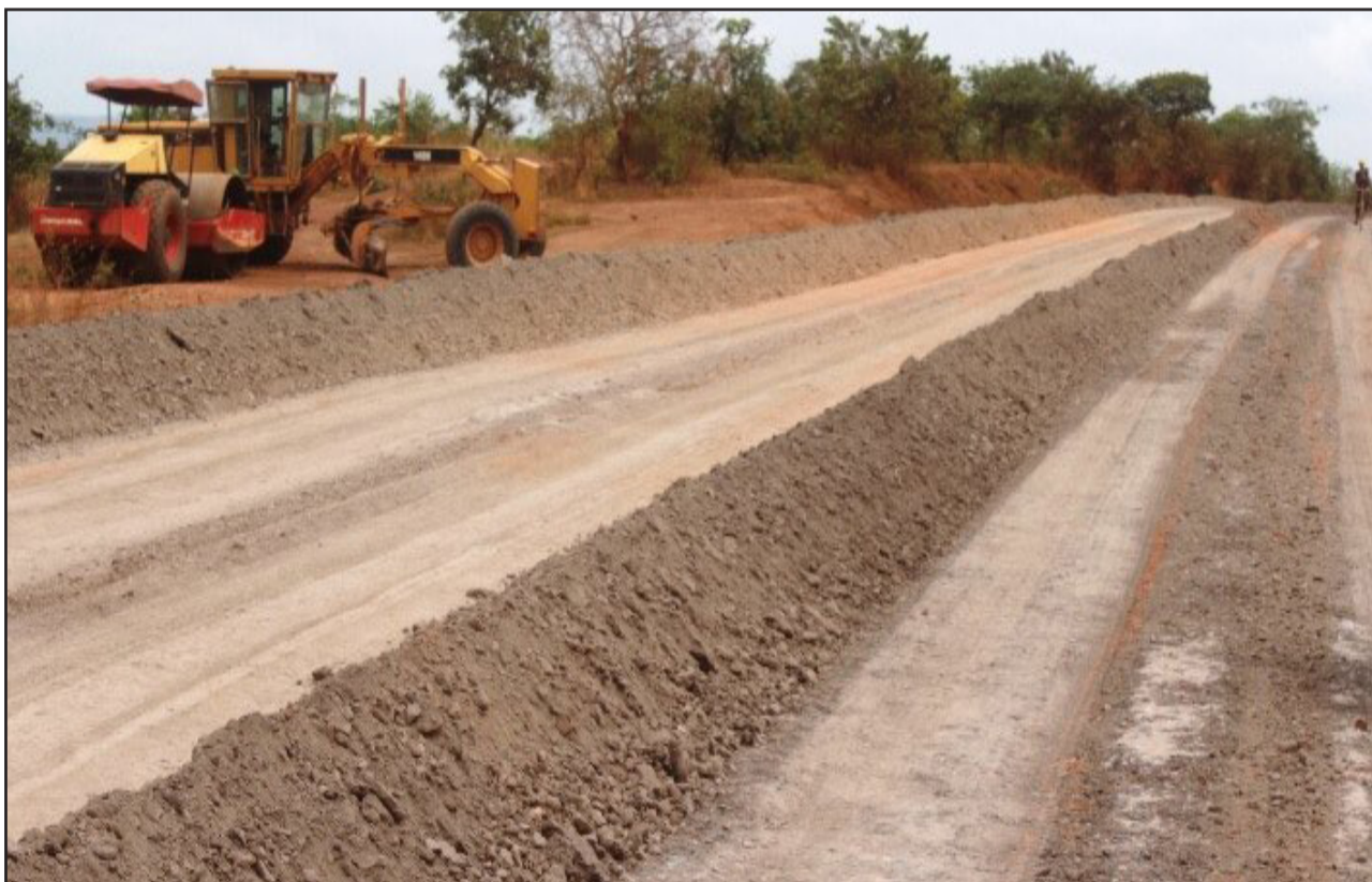
Lusahunga-Rusumo road construction in progress (Photo: Daily News)
